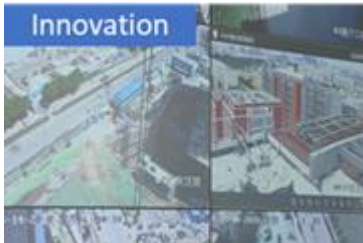
Beijing launches first 5G construction site with smart glasses and heart monitors By Global Construction Review
