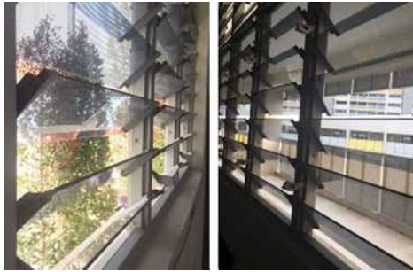
Louvers inclined at 45° to the horizontal (left), louvers inclined at 135° to the horizontal (right).
