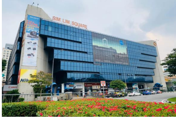
Building: Sim Lim Square Solution provider: Ampotech Pte Ltd
