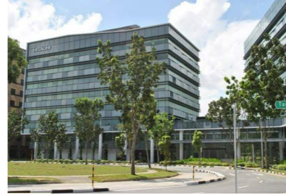
Building: Tampines Grande Solution provider: Hitachi Asia Ltd
