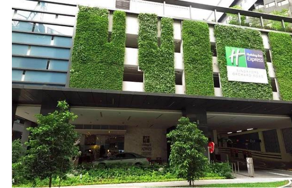
Building: Holiday Inn Express at Orchard Solution provider: Natflow Pte Ltd
