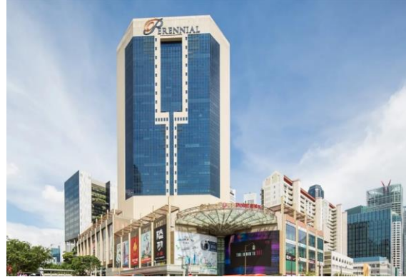
Building: Chinatown Point Solution provider: Advanced Digital Sciences Center Kaer Pte Ltd
